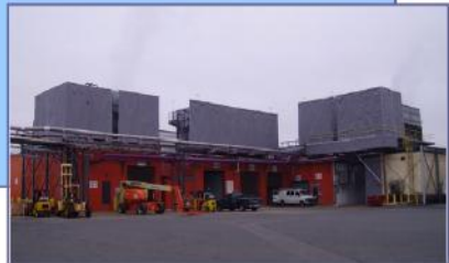
Curtain Enclosures and Barrier Walls
