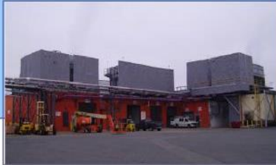
Curtain Enclosures and Barrier Walls Enclosures
