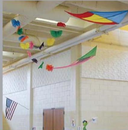
Elementary school's multipurpose room has ArtEx® One Panels installed to improve learning environment
