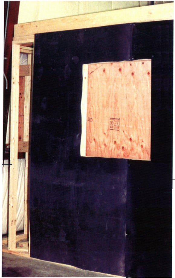
B-10 NR attached to studs before drywall is installed will significantly reduce noise transmission between rooms.
